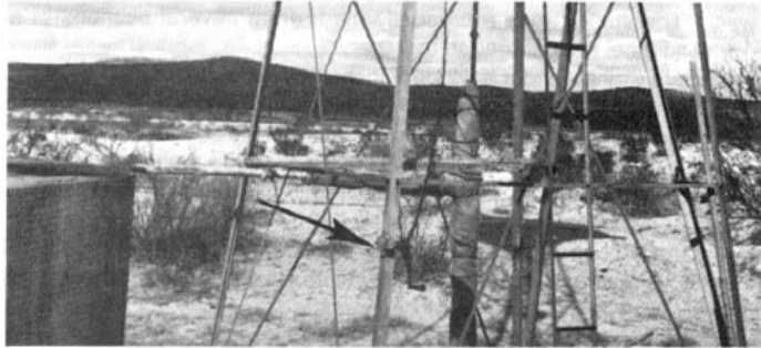
Windmill. Note windlass (arrow).
